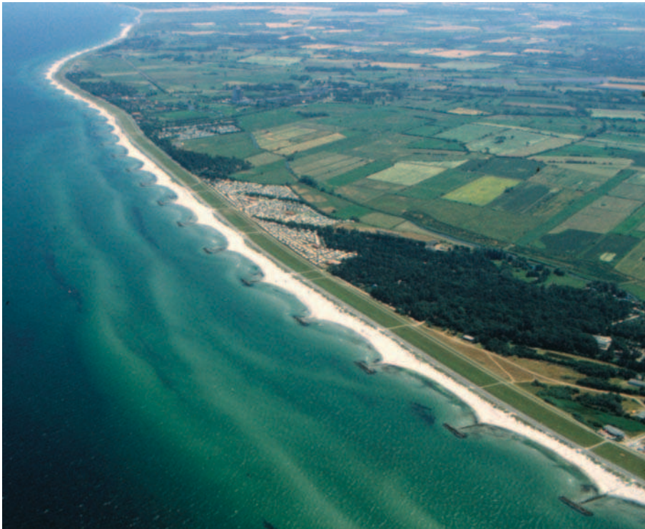
Fig. 4: State dike with T-groins about 25 km to the Northeast of Kiel
