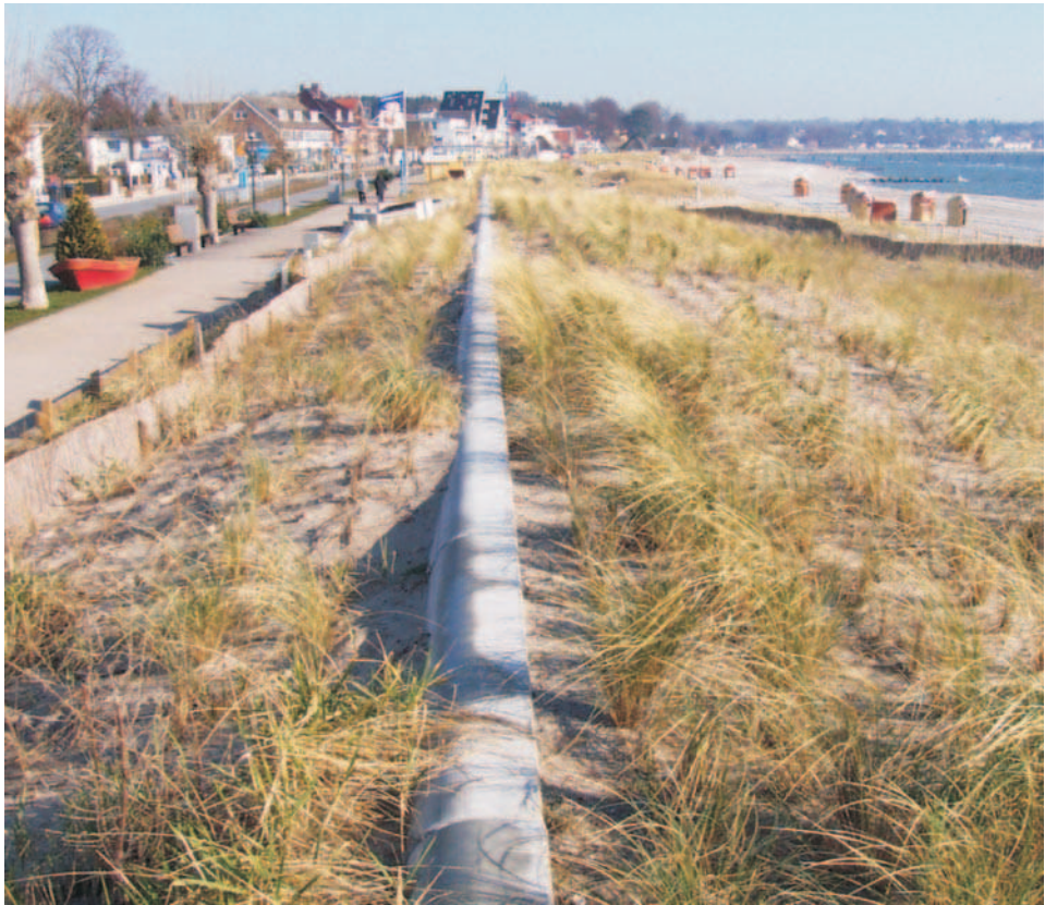
Fig. 9: Flood defence scheme “hidden” under sand and marram grass
