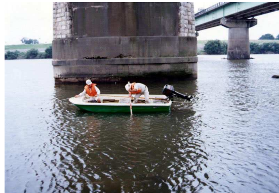
Photo 2 - Conventional investigation technique for scour from a boat
