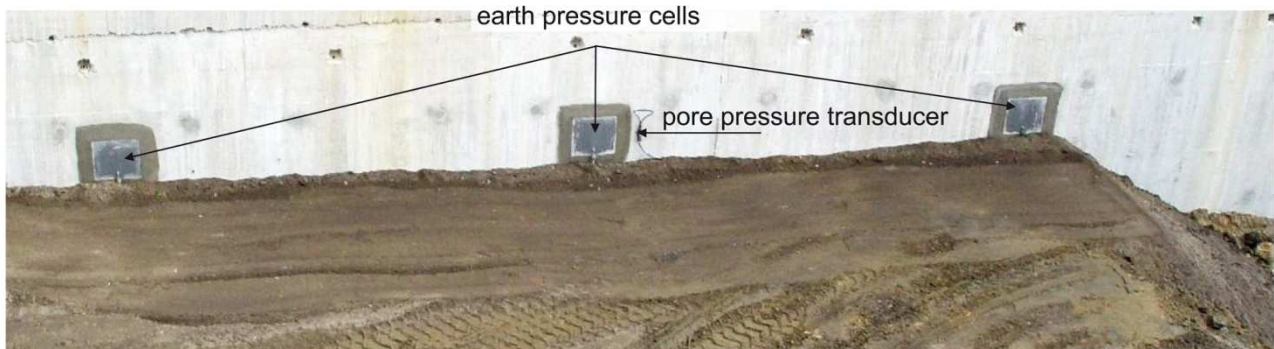
Figure 14: Installation of earth pressure cells
