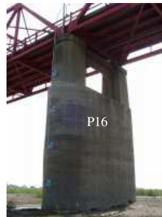
Figure 3. Completed installation of the manual-readout SMC scour monitor
