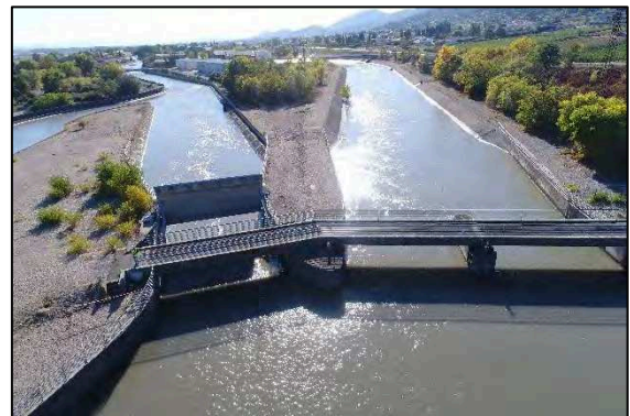
Fig. 17 Saint Saturnin diffuence (view from upstream with a drone)
