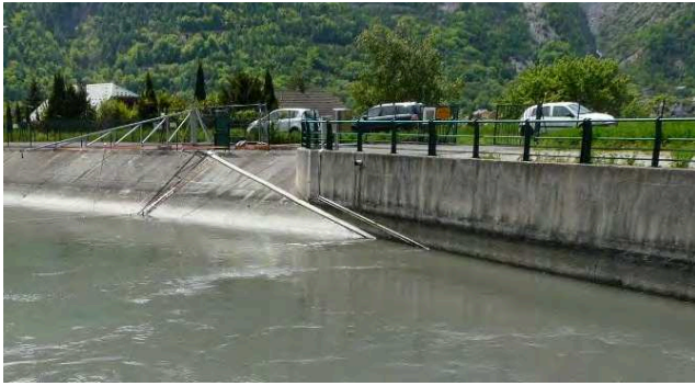
Fig. 3 Measuring flow and water level using a radar sensor at the downstream extremity of the channel
