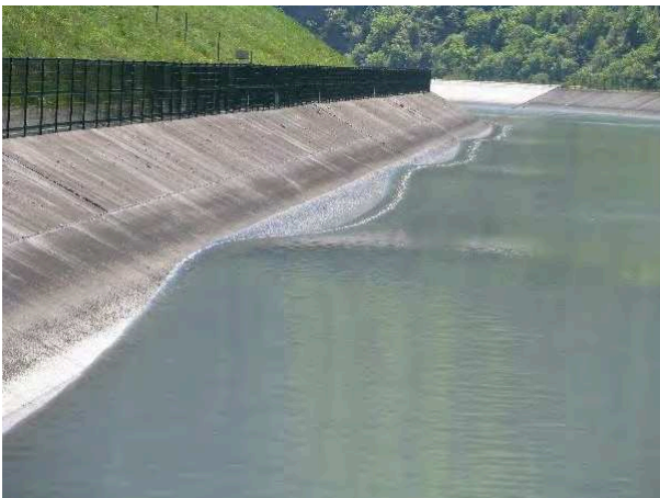
Fig. 4 Wave propagation going to the upstream, observed during the tests carried out in April 2015
