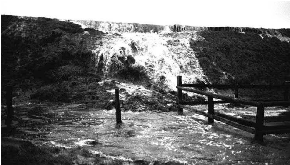
Fig. 4: Breaching dike (photo: SCHOLZ, 1976)
