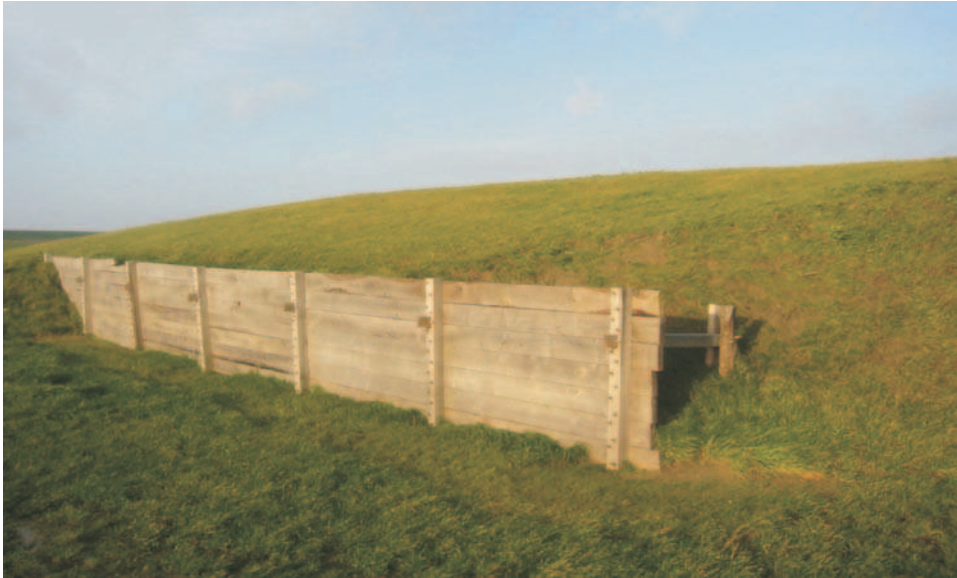
Fig. 3: Stack dike (about 1600) at the dike museum in Bösüm (photo: MEIER, 2006)
