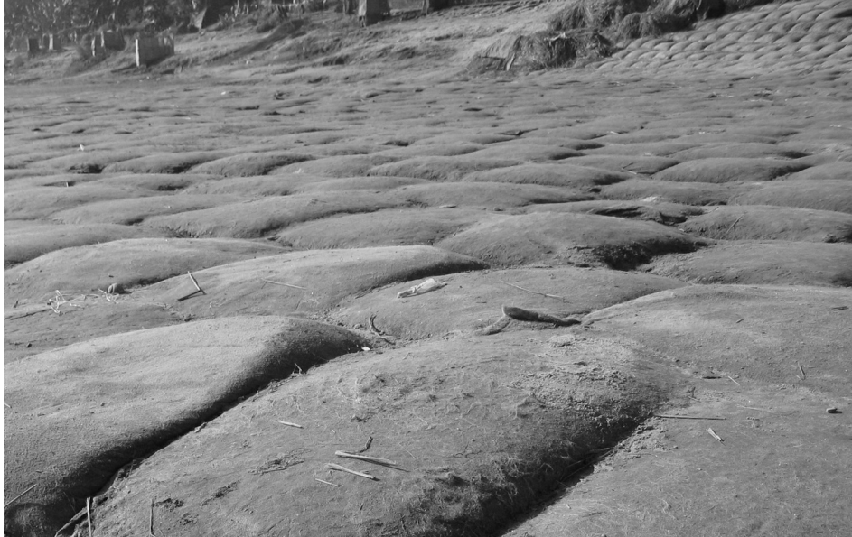
Fig. 5: Bank protection using geotextile containers (Bangladesh, courtesy K. Oberhagemann)
