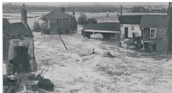
Fig. 2: Flooding in Lincshire during the 1953 storm surge
