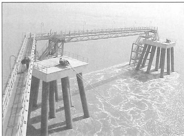
Figure 3. Tidal flow around mooring dolphins at the jetty (flow from right to left).
