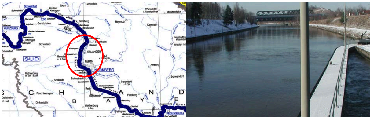
Figure 1: Location of the regarded locks (left) and situation in-situ (right)
