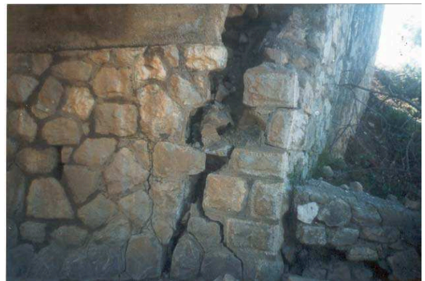
Photo nr. 6. Kallmeti bridge. It shows cracks of pillars from erosion phenomenon
