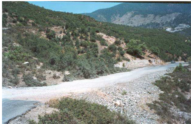
Photo nr. 8. Shkopeti landslide. It's looking to north-east, and shows, the movement of Miloti-Burreli road filled by gravels and landslide body
