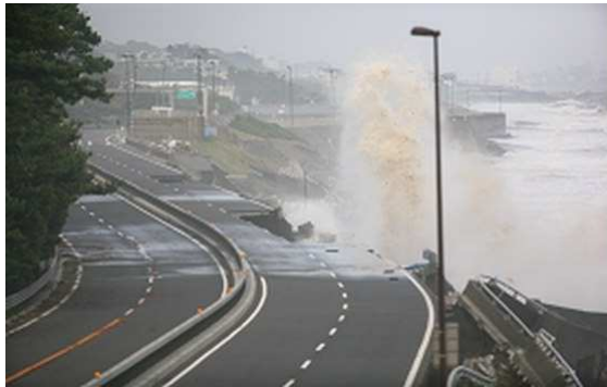
Fig.4 Waves splashing on Seisho Bypass around Ninomiya Interchange.
