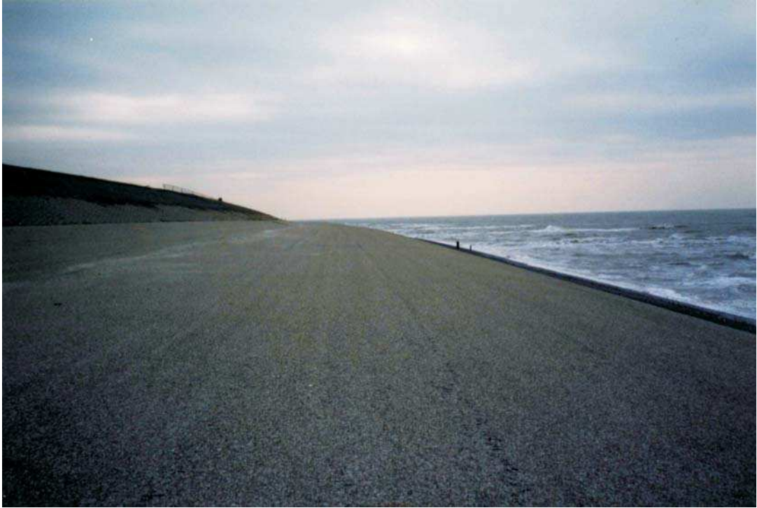
Fig. 5.16: Dike covered by asphalt (photo: SCHÜTTRUMPF)
