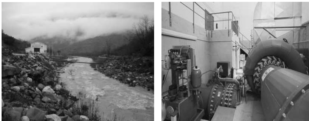
Figure 4 The power house of the Small Hydro Station Perivoli II and one of the two Francis turbines
