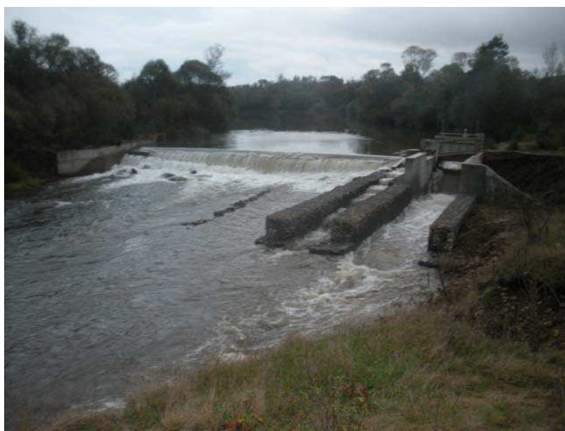
Figure 3 Installation site view after reconstruction of the existing facilities
