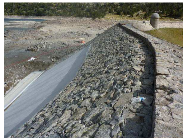
Figure 15 and Figure 16 Left: riprap being laid over the protective geotextile layer. Right: close up of completed riprap.
