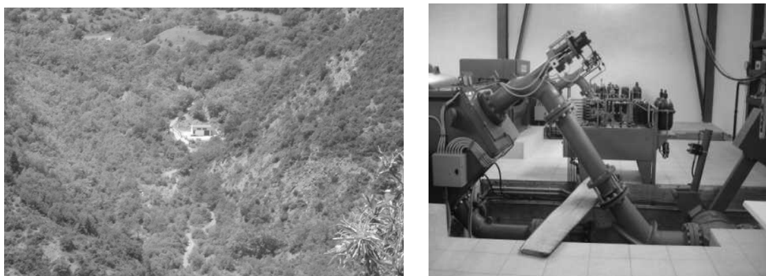
Figure 5 A general view of the site of the Small Hydropower Plant of Pougakia, with one of the two similar Pelton turbines
