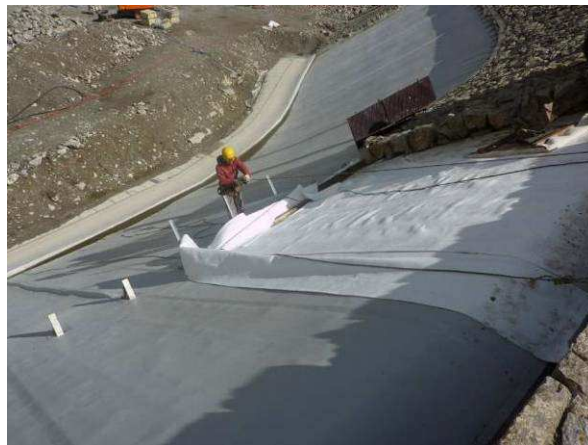
Figure 13 and Figure 14 Left: L-shaped steel brackets are installed at 2147.7m elevation. Right: a layer of geotextile is placed over the geocomposite.
