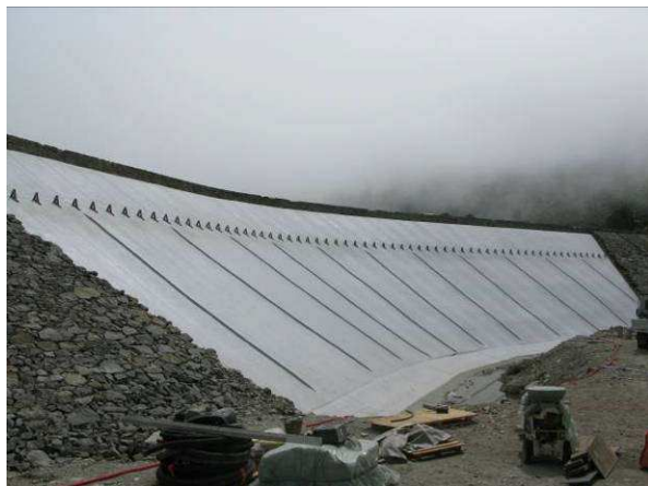
Figure 13 and Figure 14 Left: L-shaped steel brackets are installed at 2147.7m elevation. Right: a layer of geotextile is placed over the geocomposite.
