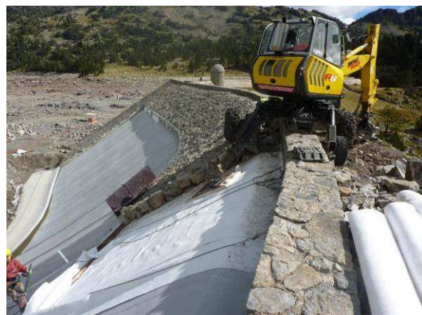
Figure 15 and Figure 16 Left: riprap being laid over the protective geotextile layer. Right: close up of completed riprap.
