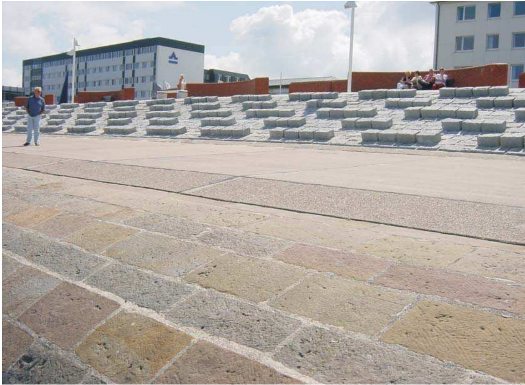
Fig. 5.19: Example for roughness elements (photo: SCHÜTTRUMPF)
