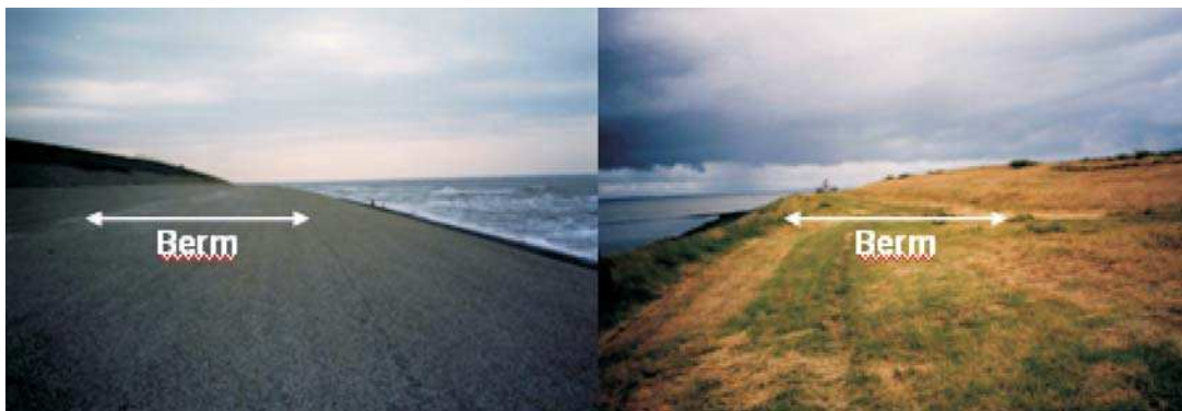
Fig. 5.28: Typical berms (photo: SCHÜTTRUMPF)
