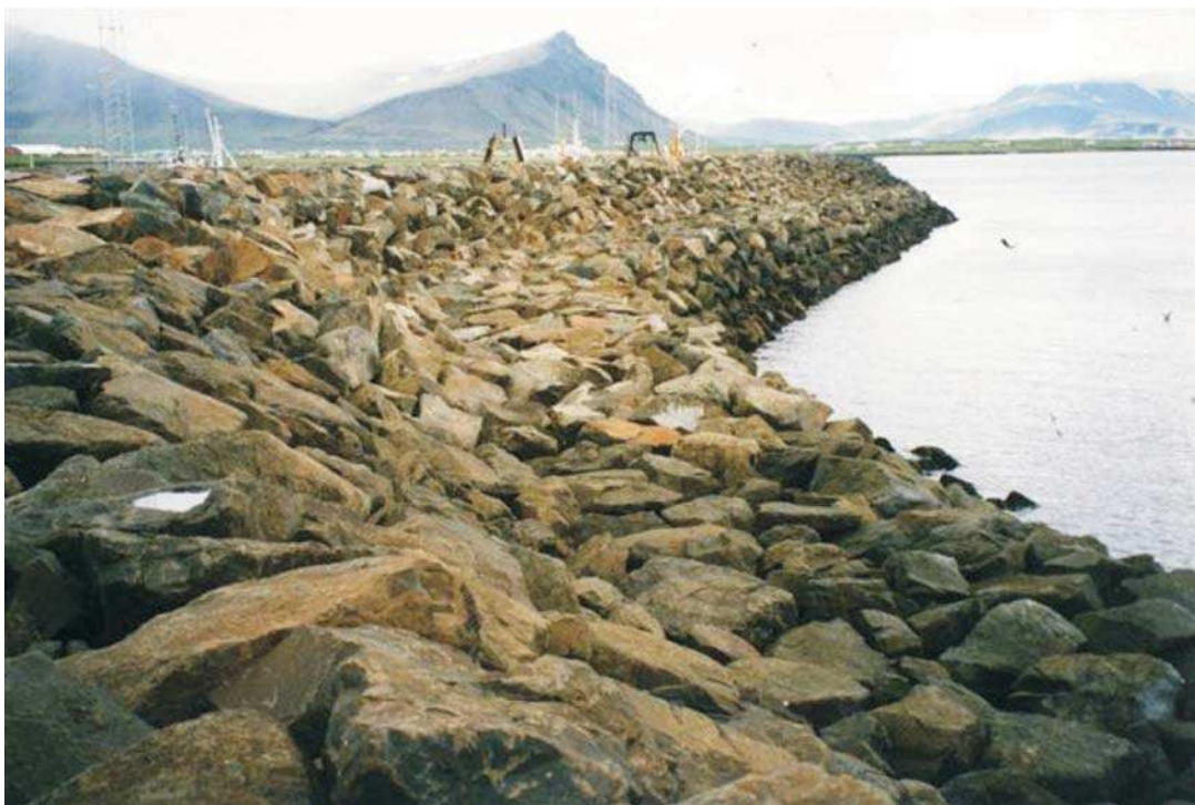
Fig. 6.7: Icelandic Berm breakwater
