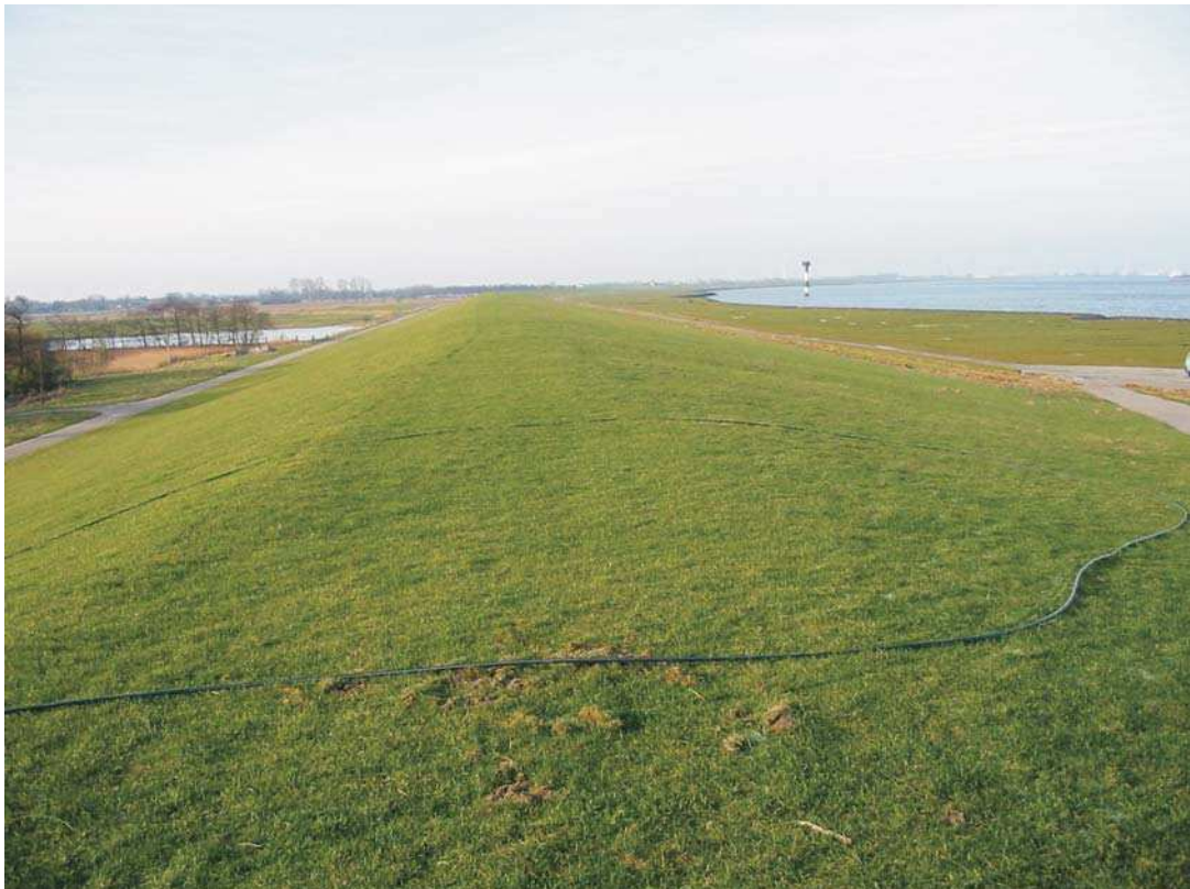
Fig. 5.15: Dike covered by grass (photo: SCHÜTTRUMPF)
