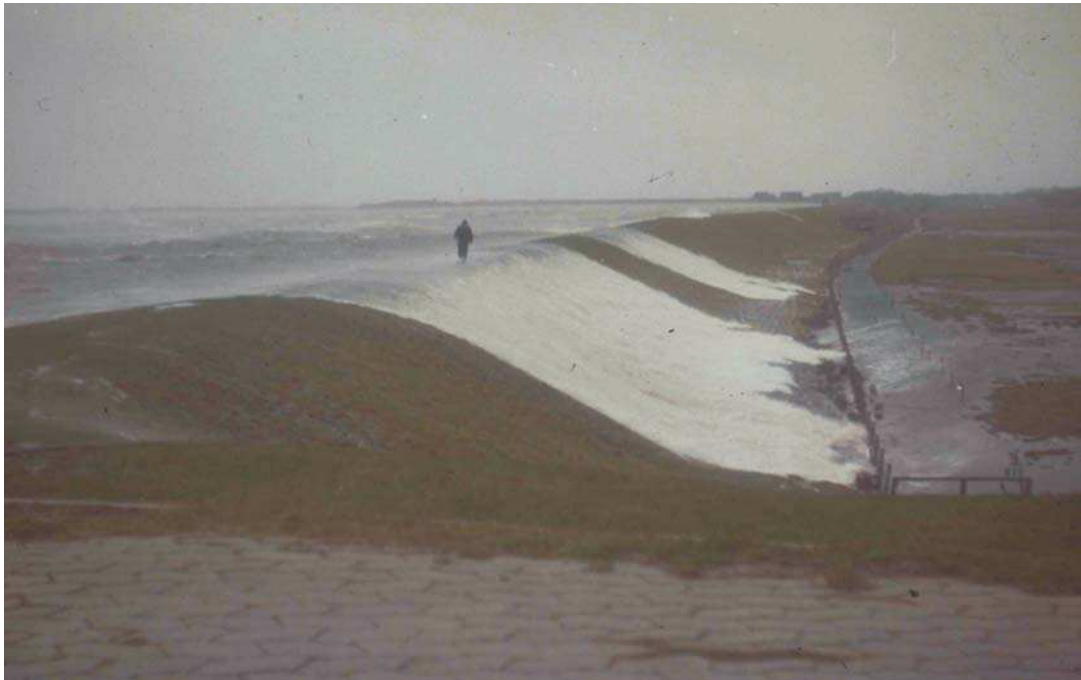
Fig. 5.33: Wave overtopping on the landward side of a seadike (photo: ZITSCHER)
