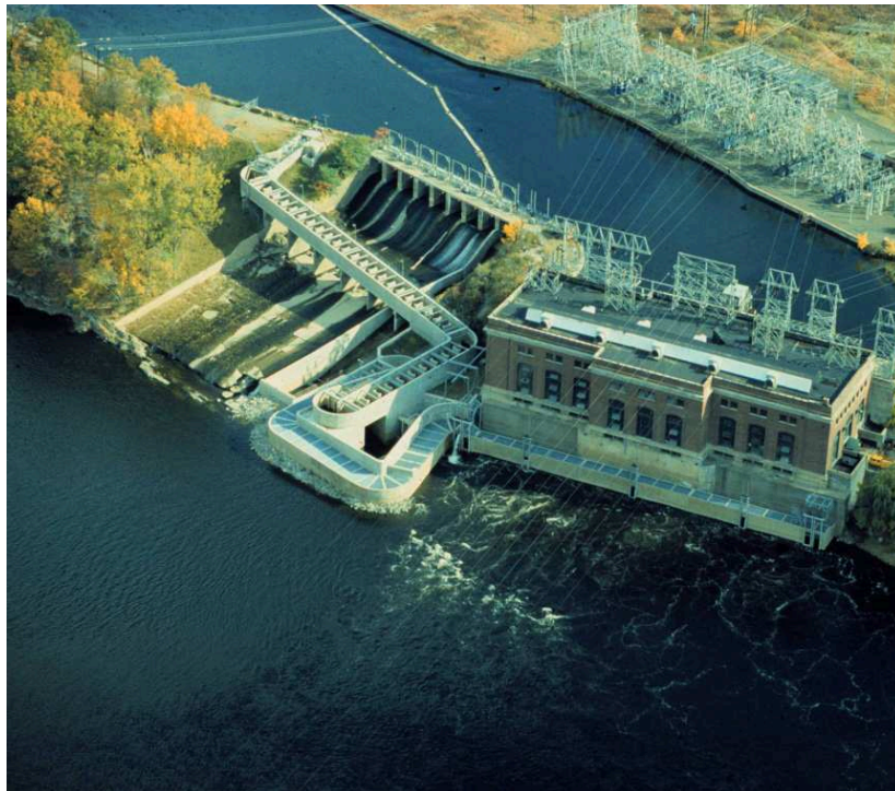
Figure 3: Cabot fishway, RKm 194 on the Connecticut River, Massachusetts USA. Constructed in 1980, this fishway has probably never passed shad effectively.
