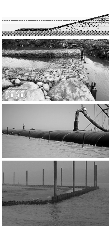
Figure 4: Construction types for the bordering dam
