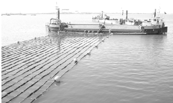
Figure 6: Geotextile layer before controlled sinking process
