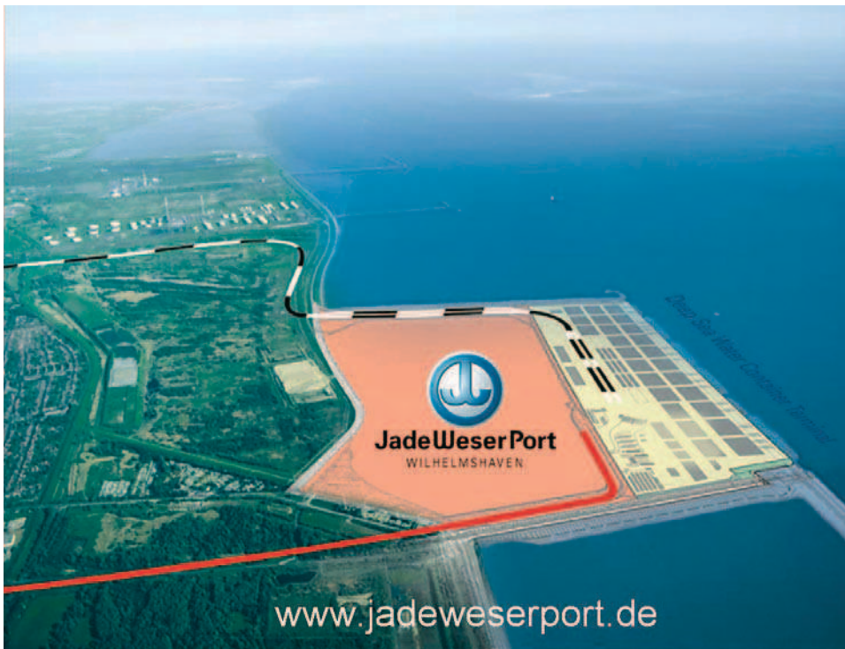
Fig. 9: Joint project Jade-Weser-Port
