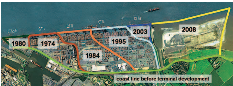
Fig. 3: Development stages of Container Terminal Bremerhaven
