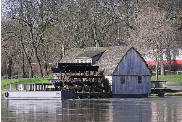
Fig. 2: Typical floating mills (a) Floating mills at Cologne / Rhine, 1856 (b) Replica mill (Rhine, 2008)
