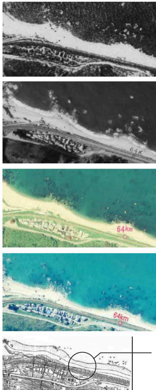
Figure 6 The aerial photographs and plane diagram in and around the collapse site.
