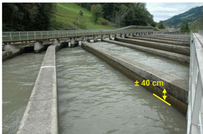
Figure 3. Prototype with water surface swinging up and down.
