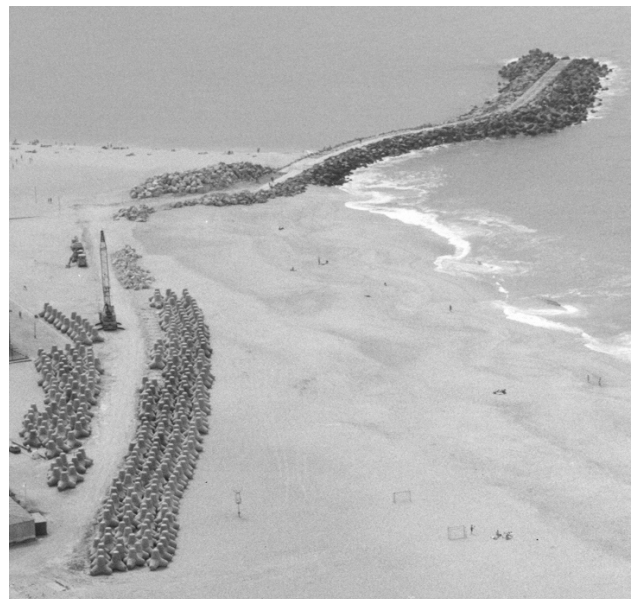
Figure 7. Reconstruction of the North groin of Espinho, 1997.
