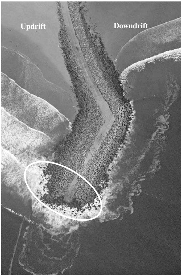
Figure 9. Central groin of Espinho, 2005.
