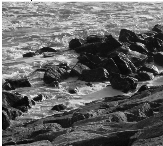
Figure 15. Toe berm of a groin at Costa Nova, 2003.
