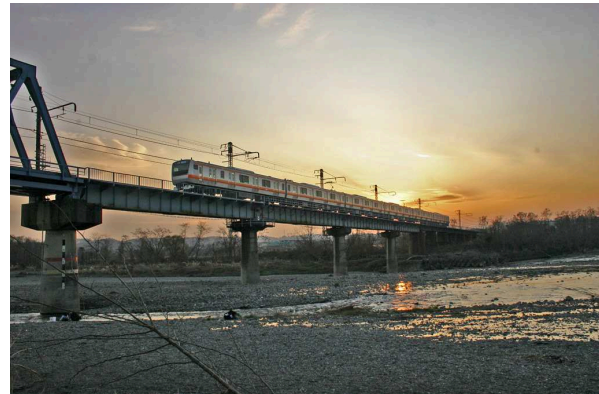
Fig.1 The view of bridge A
