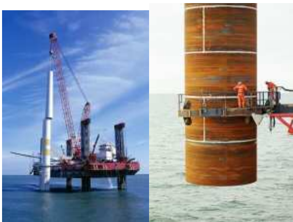
Figure 12. Installation of wind turbines at Arklow. © Airtricity
