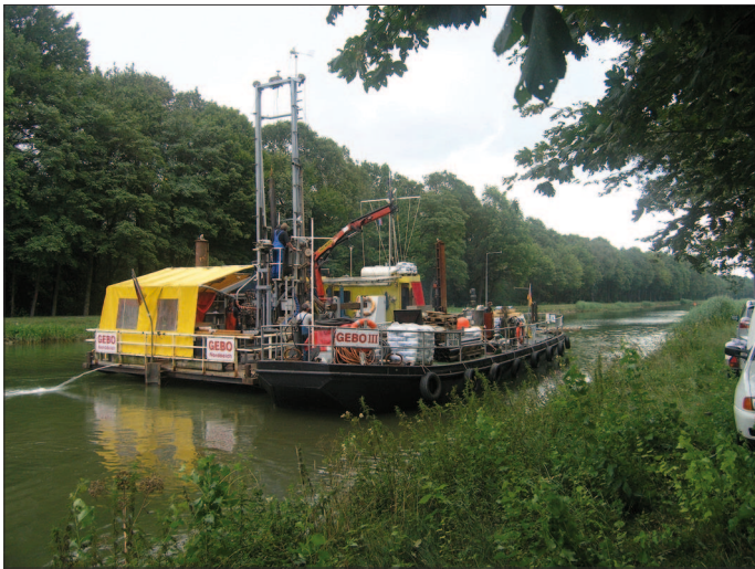
Bild 2.2: Bohrarbeiten am DEK-Nord Figure 2.2: Drilling work at the DEK (north)
