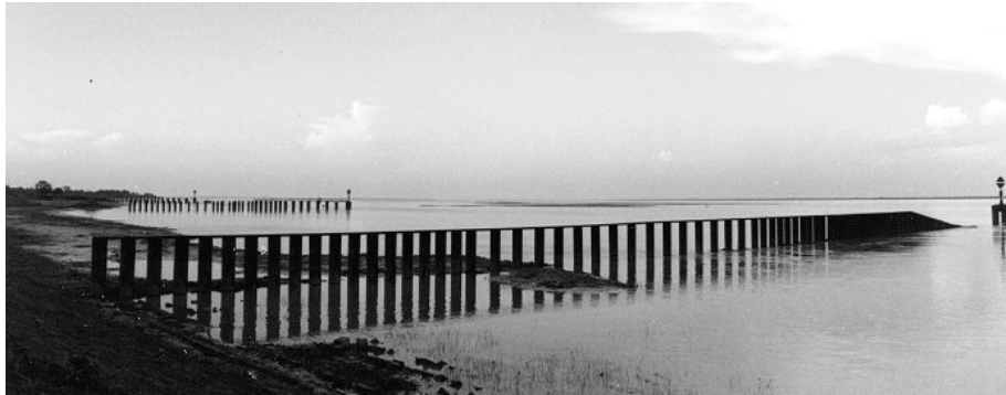
Figure 8. Permeable spurs at Kamarjani.
