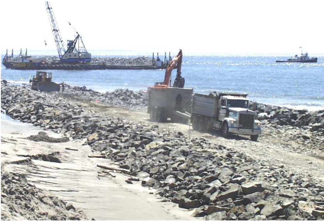
Figure 5. Project During Construction
