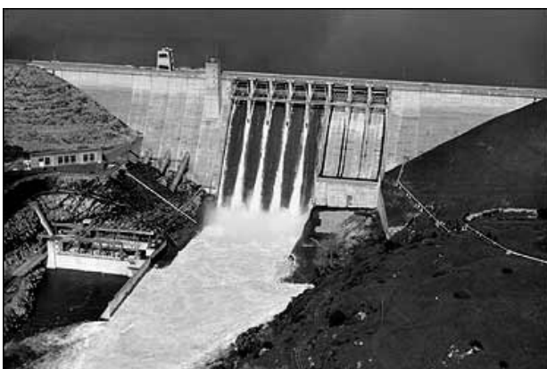
a) General view of dam and stilling basin
