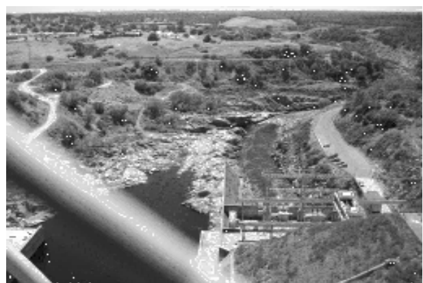
b) Downstream view of stilling basin and channel
