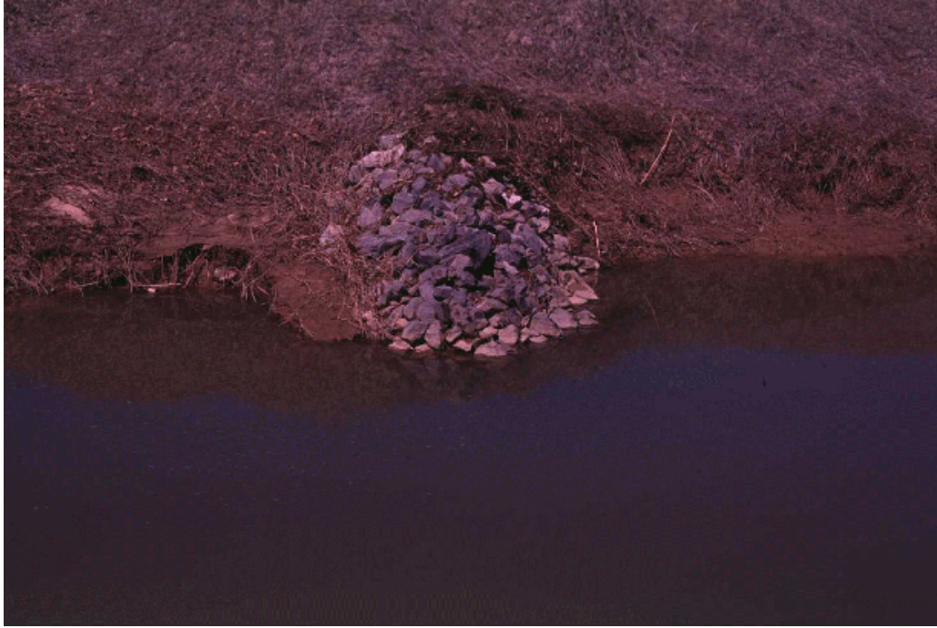
Fig. 5. Spur dike on Goodwin Creek Experimental Watershed, Mississippi. Flow direction is from right to left.
