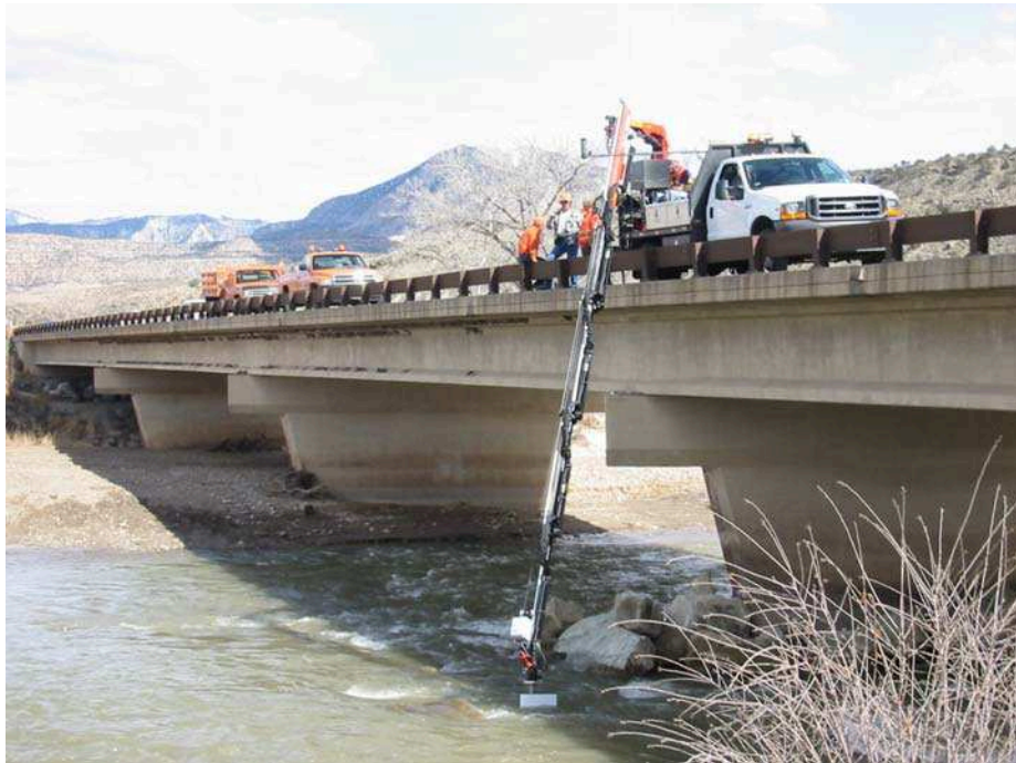
Figure 11. Truck mounted articulated arm with sonic transducer, fathometer, and computer.
