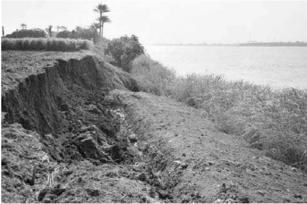
Figure 11 Bank erosion near Beni Suef (Nile main branch)
