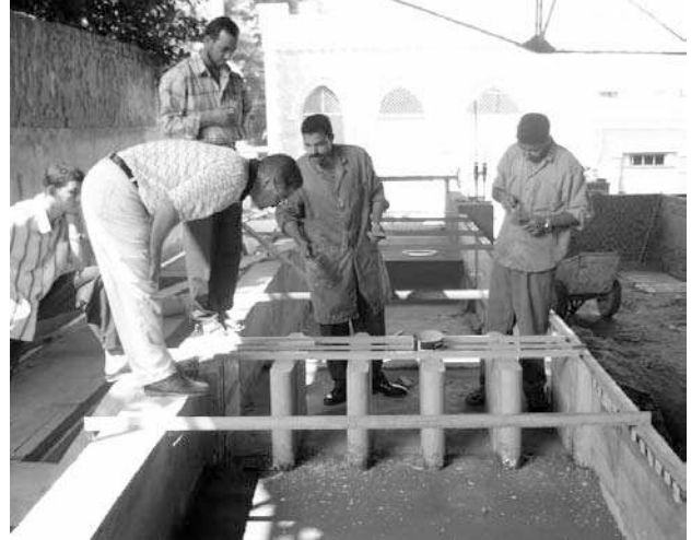
Figure 9 Scale model test for Rosetta Barrage: construction of the model at HRI
