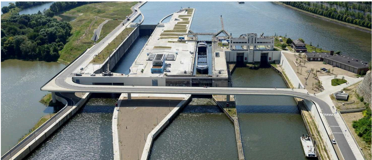
Fig.7: Downstream view – new bridge – © JL DERU/photo-daylight
