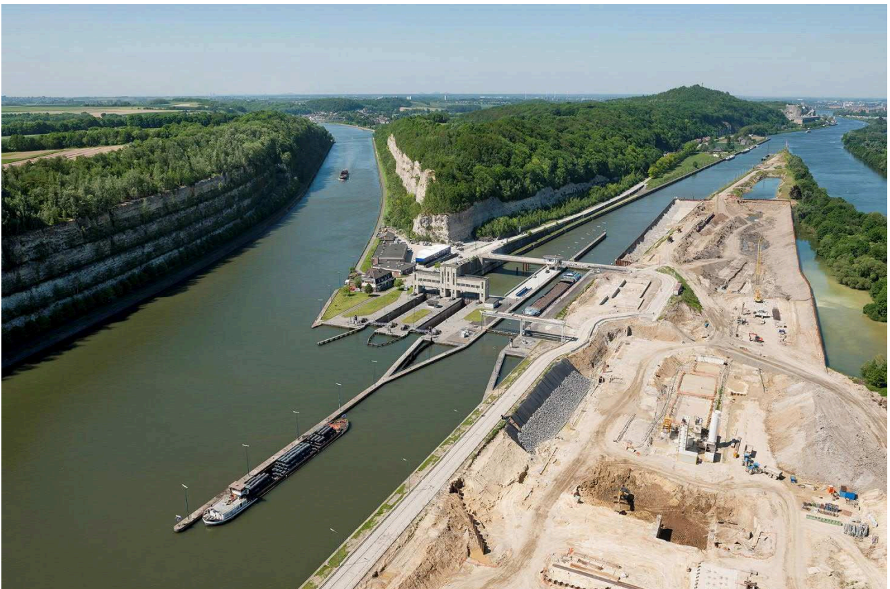
Fig.8: Overall view during excavations– © JL DERU/photo-daylight
