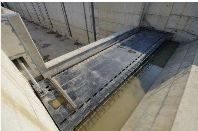
Fig.5: Upstream flap gate – © Greisch
