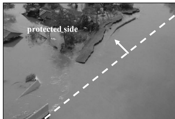
Figure 9. Stability failure in New Orleans due to hurricane Katrina (modified after ILIT, 2006)
