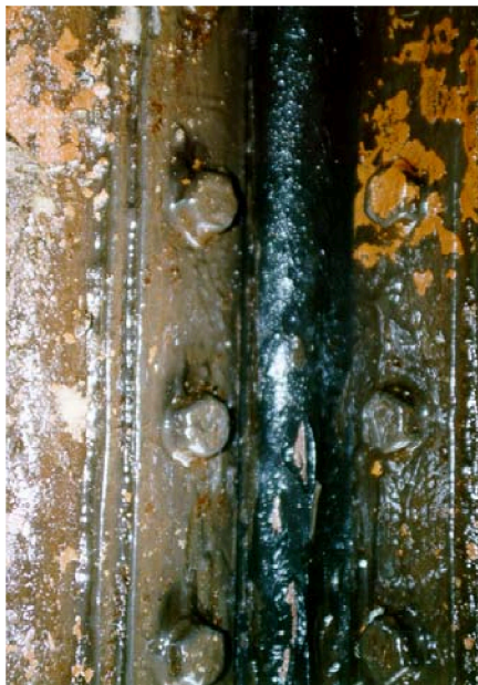
Pic. 2: damage of a waterstop
