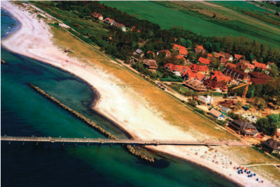
Fig. 3: Breakwaters and sea bridge in Wustrow
