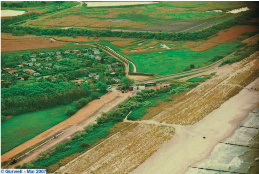
Fig. 5: Groynes, beach nourishment, dyke and steel wall in Markgrafeneheide
