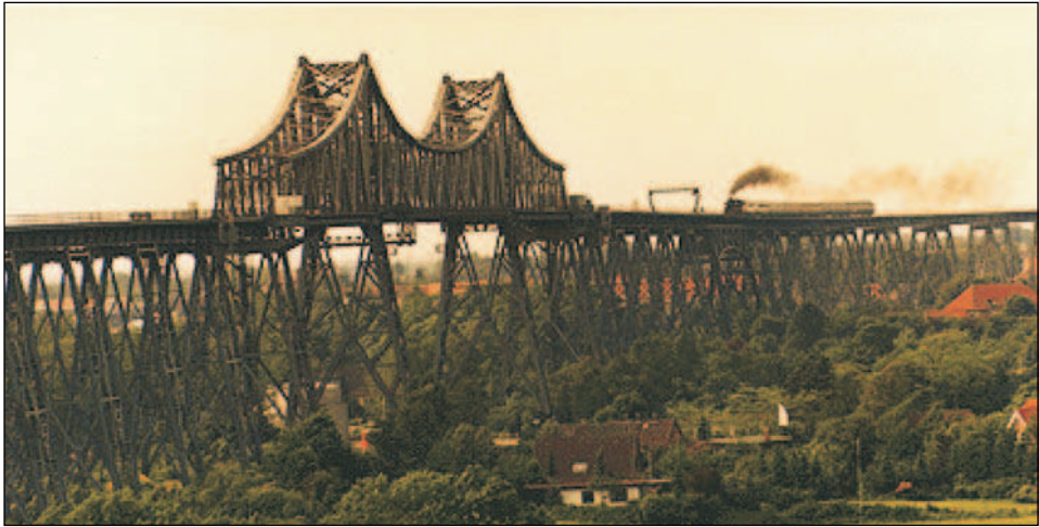
Fig. 8: Elevated railway bridge (STADT RENDSBURG, 2008)
