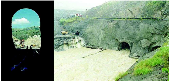
Figure 10: Interior view of tunnel entrance and flood passing at exit
