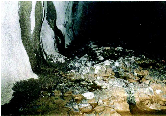
Figure 11: Unlined rock floor of tunnel after flood, remaining essentially intact
