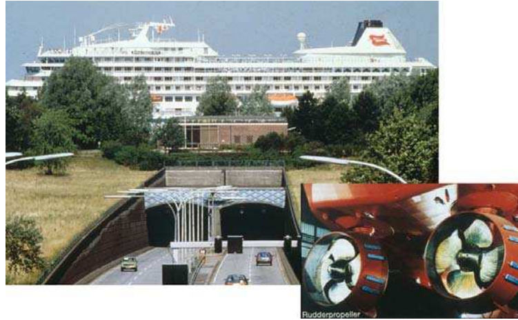
Figure 2. The road tunnel under the Ciel canal - the propellers of the vessel are producing a turbulent flow to the embankment.
