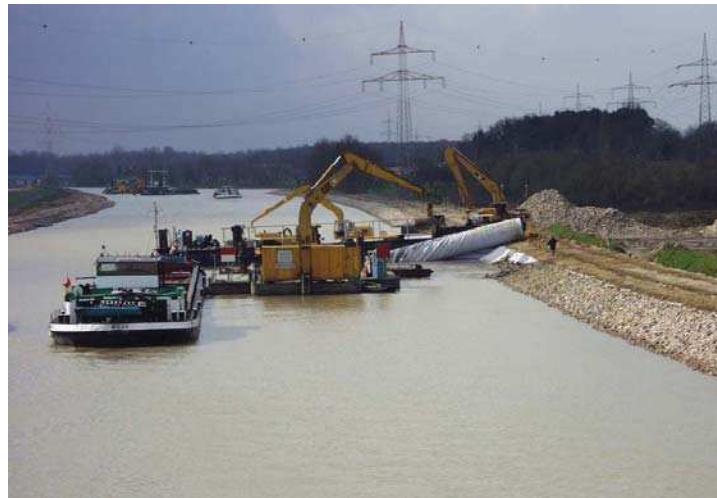
Figure 3. Geotextile installation in a navigable waterway during the passage of vessels.
