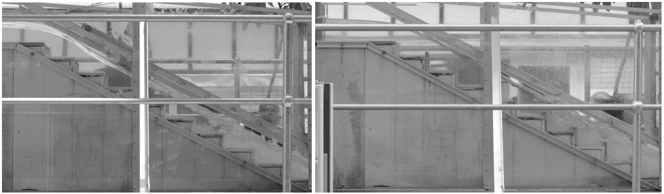
Figure 3. Skimming flow regime on flat and pooled stepped spillways - Left: flat steps, Q = 0.114 \text{ m}^3/\text{s} , d_c/h = 1.7 , Re = 8.8 \times 10^5 ; Right: pooled steps, Q = 0.100 \text{ m}^3/\text{s} , d_c/h = 1.56 , Re = 7.7 \times 10^5
