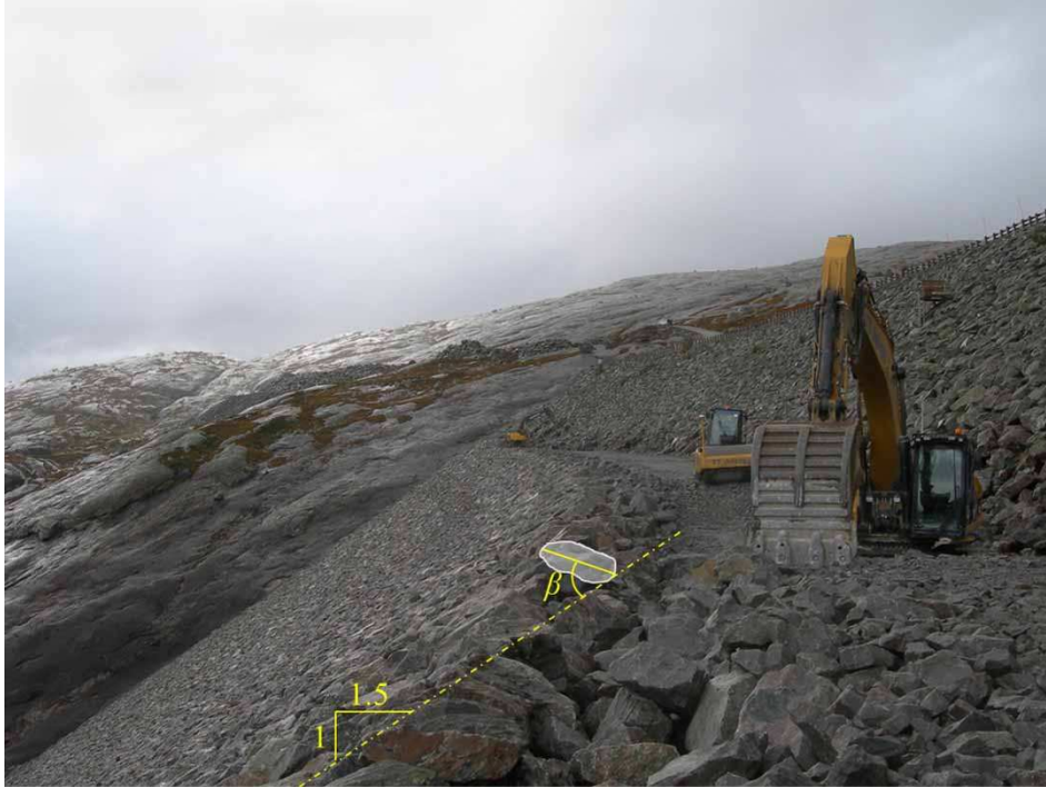
Figure 1. Rehabilitation work on the 129 m high dam Svartevatn in Norway. The riprap stones on the downstream slope are placed one by one in an interlocking pattern with their longest axes inclined towards the dam. The inclination angle \beta is the angle between the longest axis of a stone and the slope as indicated in the picture. (Photo NTNU).
