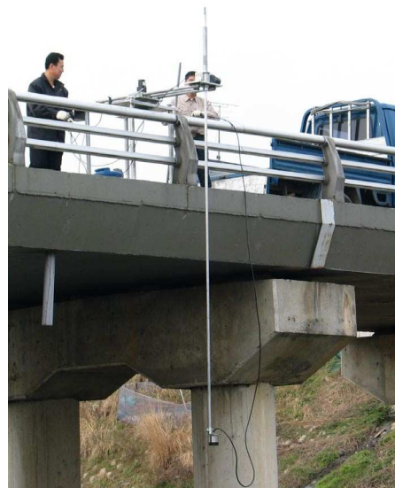
Figure 5. Scene of preparation for measuring pier scour
