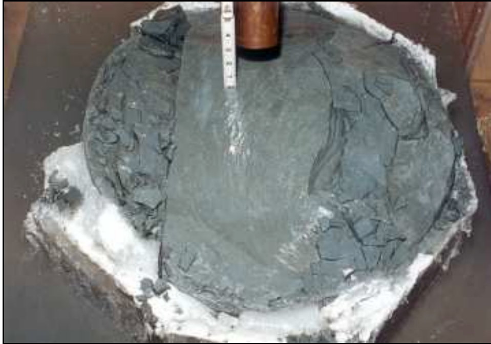
Figure 7. Undisturbed shale surface after removing deteriorated material (EXT1)
