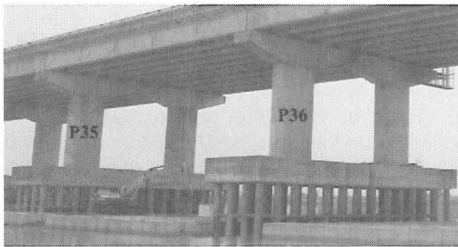
April 2009 (piles exposed around 4.5m)
