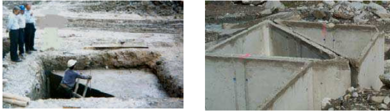
Figure 8: Prisms construction methods, without using sides' formwork and reinforcement (left), precast formwork filled with mass concrete (right)
