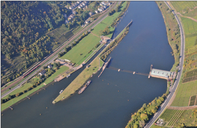
Bild 2: Einachsige Staustufe (WSD SW) Figure 2: Single-axis barrage (Waterways and Shipping Directorate South-West)
