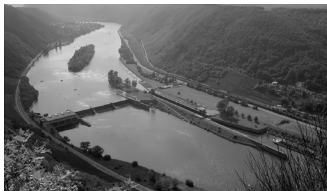
Figure 1. Barrage Lehmen with power plant, weir and ship lock at federal waterway Mosel
