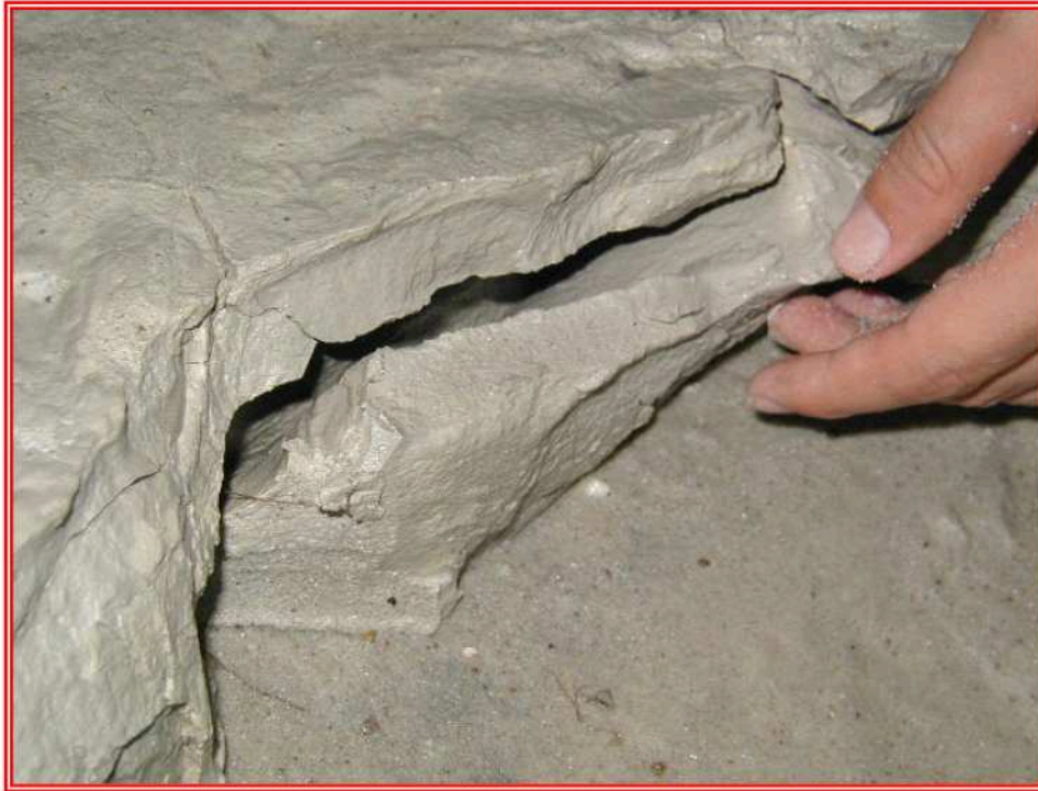
FIG 21 Falling Clay Block in the Scour Hole for Test 6
