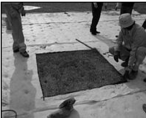
Figure 13. Extraction of samples for laboratory testing
