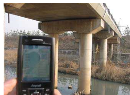
Fig.10 Photo showing the proposed bridge scour field inspection in operation
