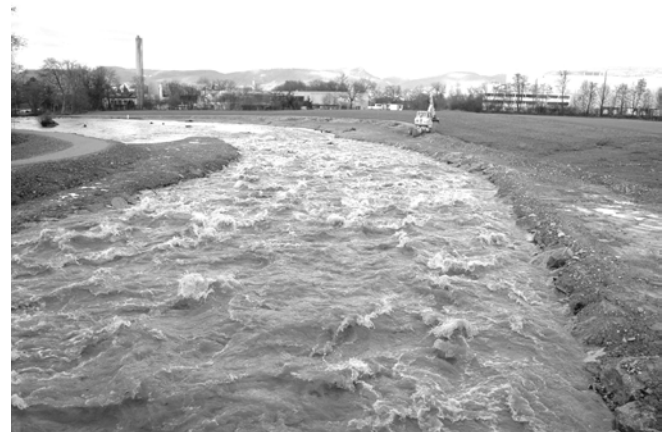
Figure 3: Downstream view of an unstructured block ramp (Wyna River, Switzerland) under undulating flow conditions.
